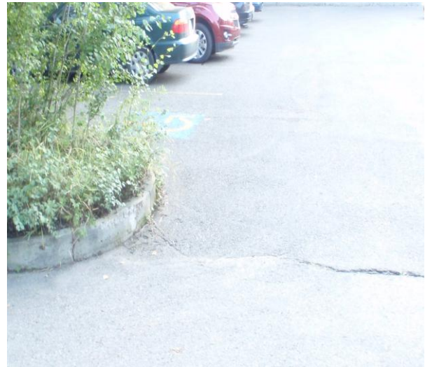
Left: A divot in the pavement and loose gravel located on the pathway near entrance to Shakespeare on the Saskatchewan.
